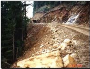
Forestry Road Construction
