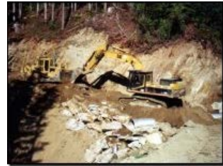
Culvert Installation
