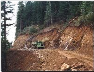
Forestry Road Construction
