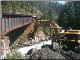
Bridge Abutment Work
