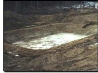
Settling Pond Construction
