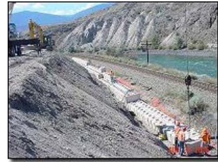
Lock Block Wall Construction
