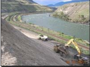
CPR Ashcroft Siding Extension
