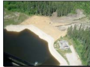
Priddis Dam Construction
