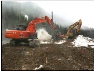
Drilling and Blasting
