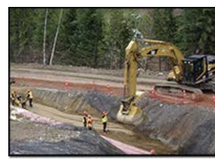
Penstock Backfill
