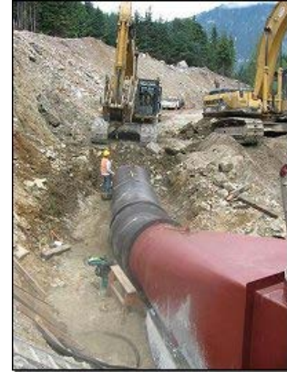
54" Ductile Iron Installation
